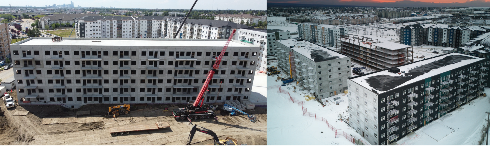
Figure 4: Installation of the 6-storey building used in this study.
