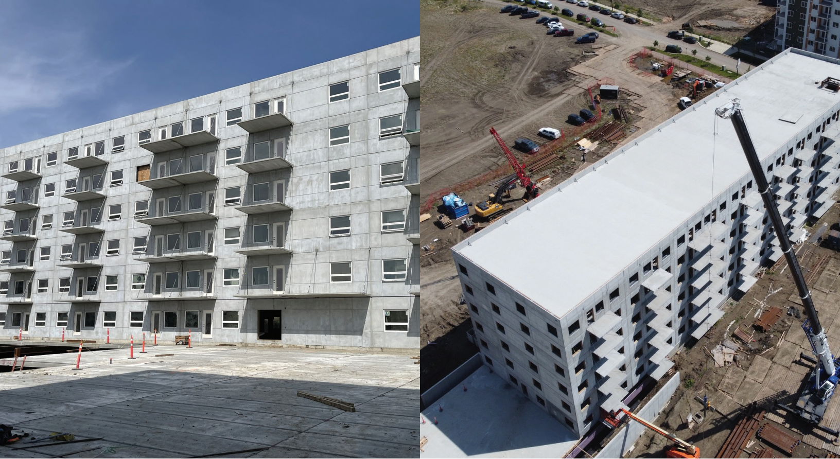
Figure 2: The 6-storey building used in this study being installed.
